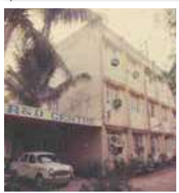
Chemical Manufacturing unit, Ambarnath, Maharashtra
