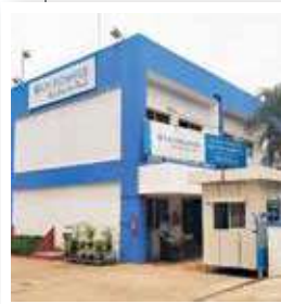
Fabrication and Assembly Unit, Hosur, Tamil Nadu
